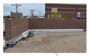
Install cricket with 1/2" per foot slope ensure proper drainage.
